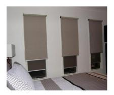
**Defect:** The blinds do not comply with the <u>mandatory safety standard for the installation of corded internal window coverings.</u>
